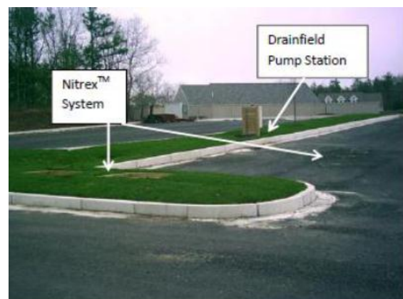
FIGURE 2-5: SMALL CLUSTER WASTEWATER SYSTEM UNDER PAVED AREA
