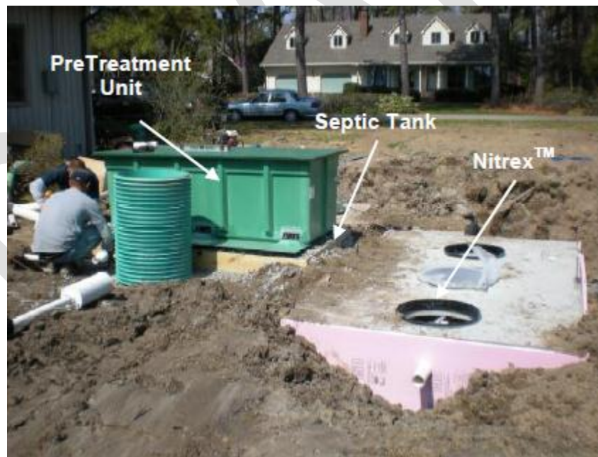
FIGURE 2-3: INDIVIDUAL PROPERTY WASTEWATER SYSTEM PRODUCING EFFLUENT TN < 10 MG/L
