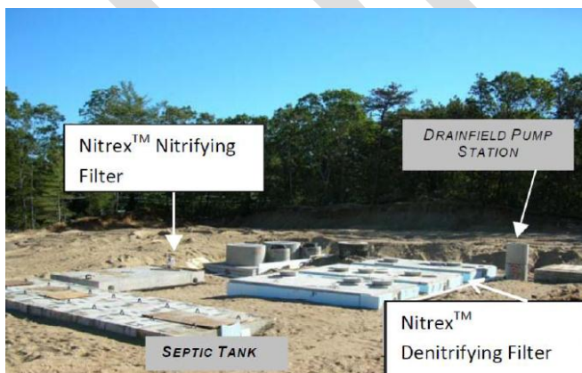
FIGURE 2-5: SMALL CLUSTER WASTEWATER SYSTEM UNDER PAVED AREA
